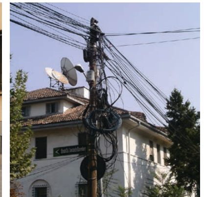
Fig. 9. Suspended wirings
