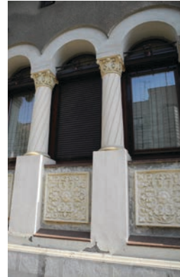
Fig. 4. Triple lancet window fitted with external metal blind.
