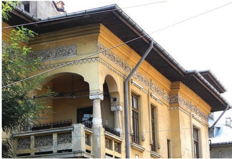
Fig. 23. The brackets under the balcony are in prefabricated elements with thin walls.
