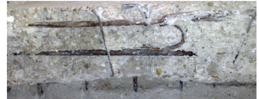
Fig.2.7 – Exposed reinforcing bars at slabs and beams
