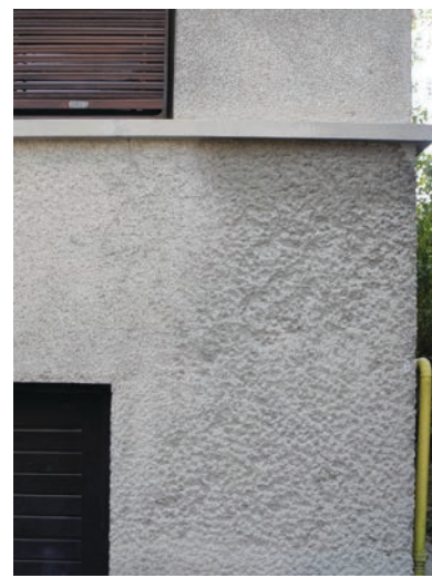
Fig.22. Two renders of different roughness are superposed, divided only by a flat fillet.
