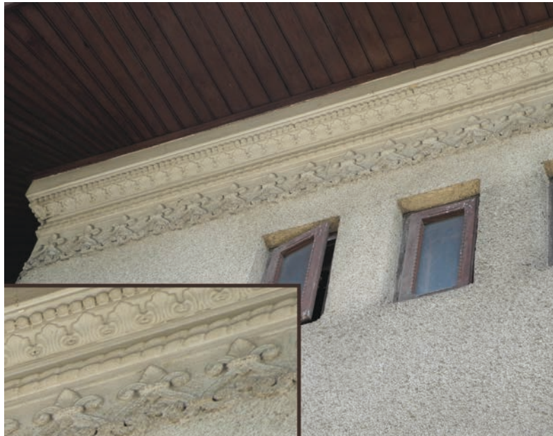
Fig.29. When making the new render, simply rough, the masons have partially covered the rich frieze at the top of the façade.
