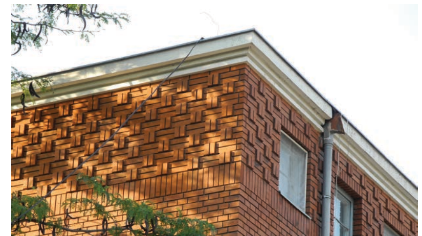
Fig. 10. The refined upper part of the Busila Villa brickwork, with the relief motif made with projecting rowlocks alternating with couples of stretchers.
