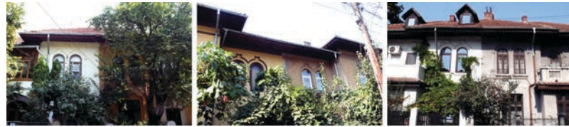
Fig. 10. The incongruous refurbishment of plasters and wall paints, concentrated on single parts of the property, alters the unitary perception of the surfaces.
