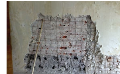
Fig.3.3 – Incoherent inner wall with old reinforcing steel mesh
