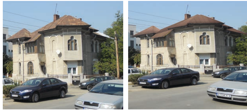
Fig. 09, 10. Bucharest, examined site. A simulation of the change of covering mantle in copper slabs (on the corner building) with an integrated solar system (to produce hot water).
