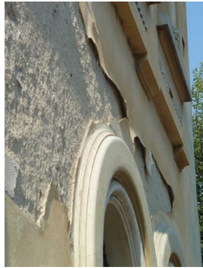
Fig. 4. Bucharest, modernist borough. An example of a villa in picturesque style with conservation problems in the outer plasters, detail (Photo R. Picone 2011)
