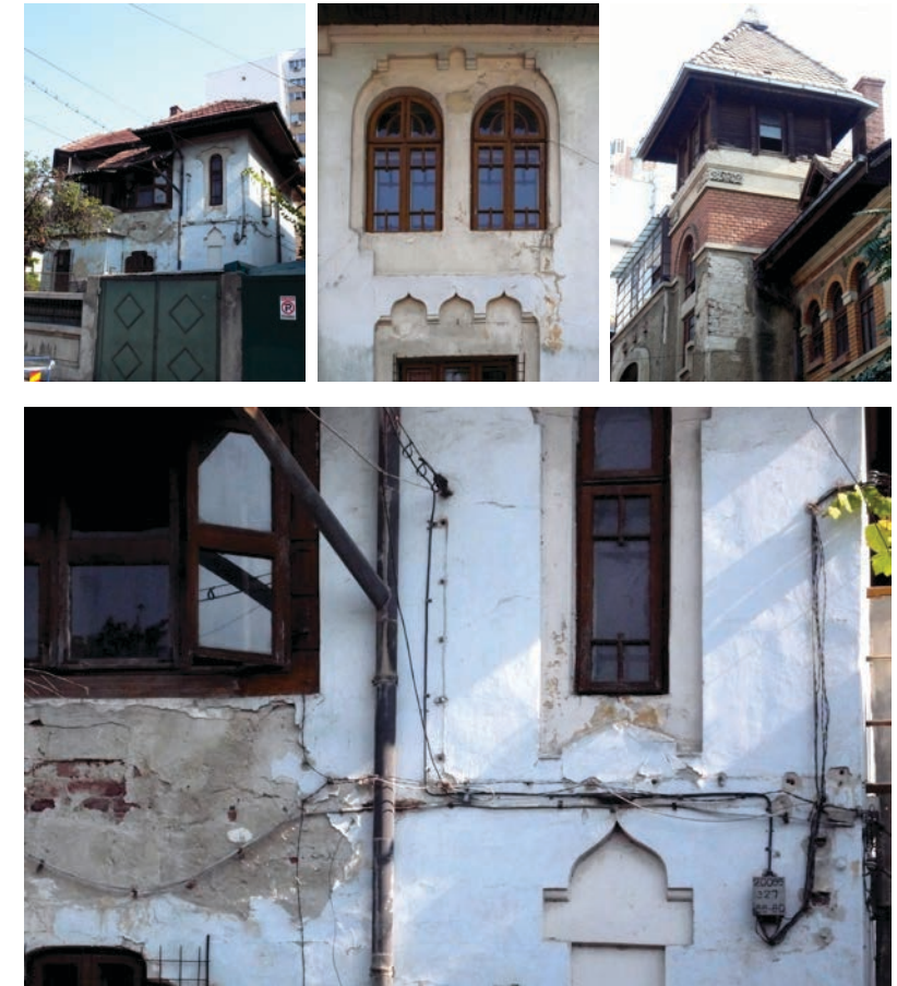
Figs. 2-5. Deterioration mechanisms of plaster surfaces and decorative elements.
