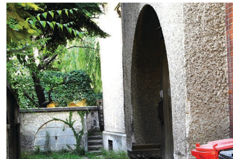
Fig. 2. The arch is supported by column capitals: in this way it was possible to place it at the height of the ground floor entrance.
