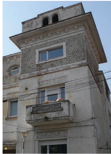
Fig.21. The rare plaster of the upper level of this building, made putting on a rough render many flashing big quantities of mortar, then flattened, with the final effect of a series of irregular flat circular shapes on a rough bottom. This upper part of the façade and the above protruding eave, a classical cornice with even dentils, has a strong contrast with the lower, smooth, part of the façade.
