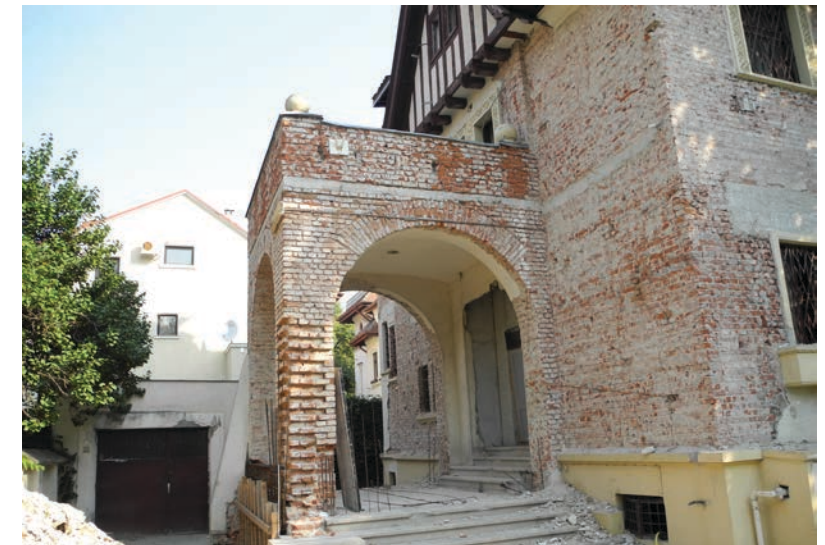
Fig.. 3. The building, scraped off plaster and decorations, shows a vertical traditional brick masonry, coupled with concrete slabs and lintels.
