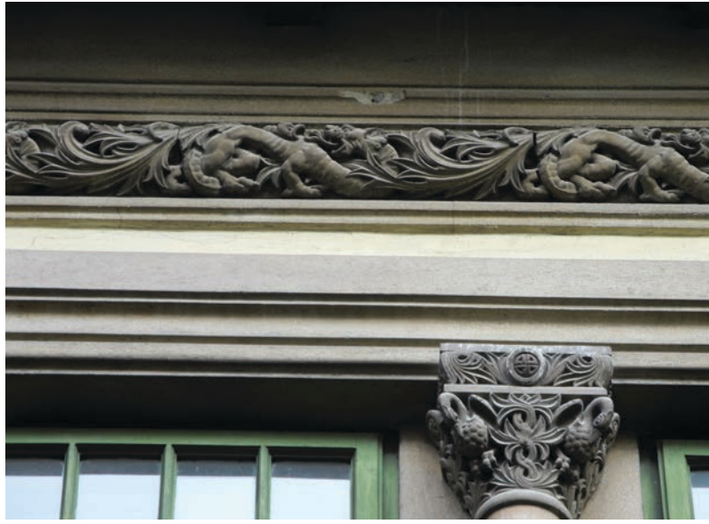
Fig. 13. The joint between prefabricated pieces is visible in the horizontal cornice.
