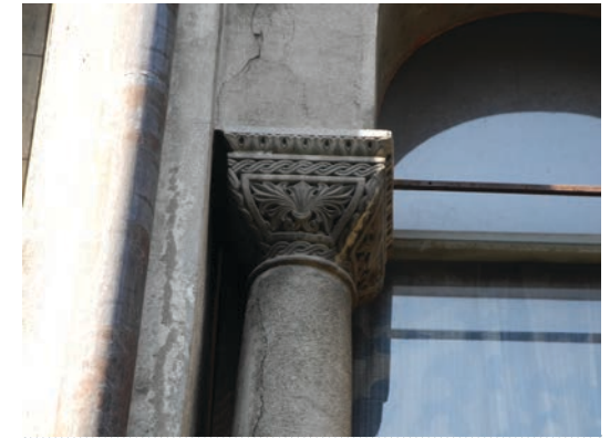
Fig.13. The cladding in artificial stone of the column and of the above arch, texturized with a bush hammer, is now detaching and appears particularly difficult to be restored.
