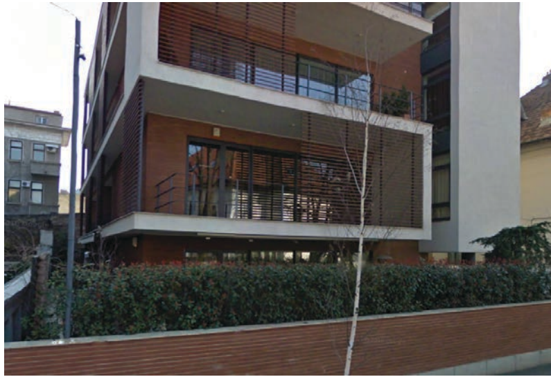
Fig. 32. Wooden diaphragms at a new building on Strada Praga.
