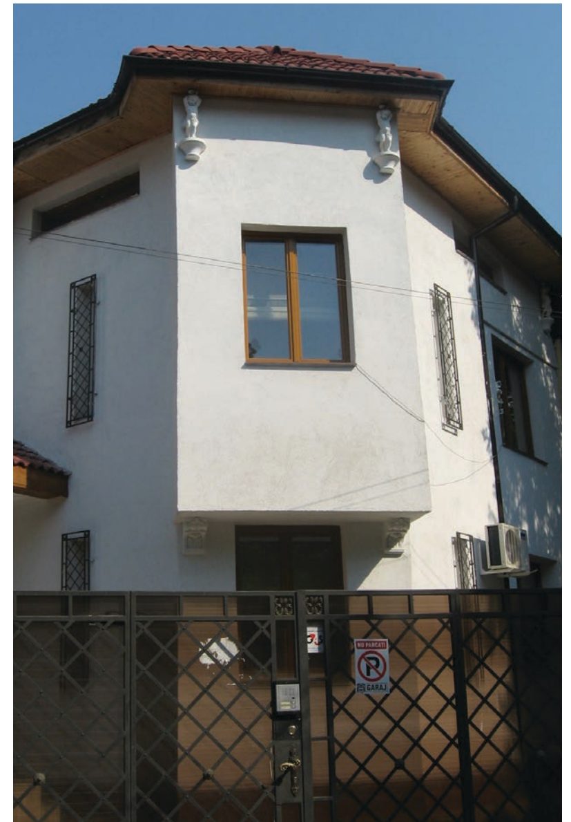
Fig. 13. Replacement of the original windows with new ones deriving from current industrial production.
