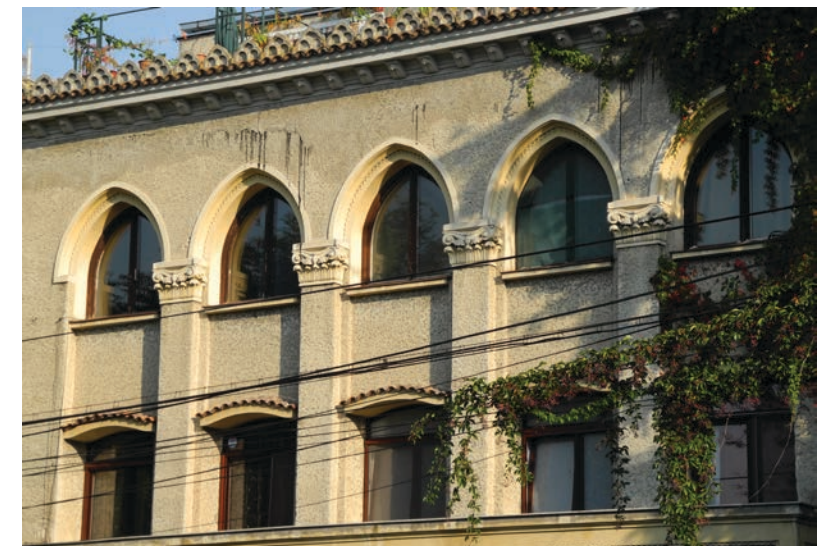
Fig.. 4. The plaster of the façade is marked by many dark drippings due to leakage of the terrace insulation over the concrete slab.
