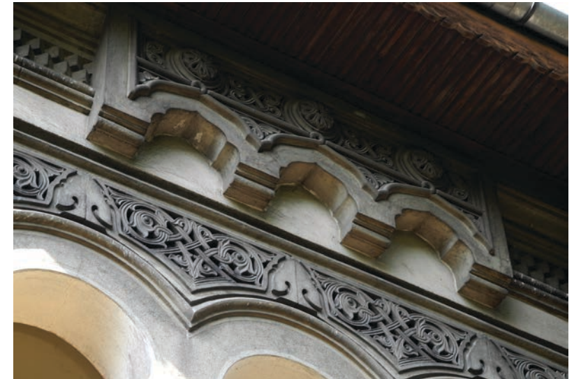
Fig. 21. Decorations made with prefabricated panels.
