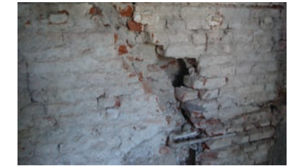
Fig.3.4 – Crack in inner wall
