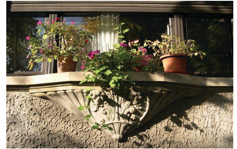
Fig.19. The particular texture of the render highlights the cast stone elements placed on it.
