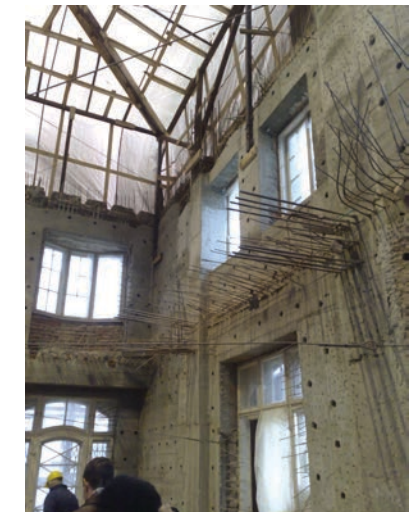
Fig.3.12 – Peripheral load bearing tube in reinforced concrete
