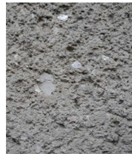
Fig. 26. The plaster with the inclusion of small shiny elements, probably of a micaceous nature.
