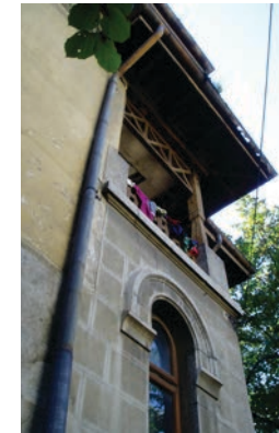
Fig.12. The false ashlars in artificial stone of a façade in traditional Romanian style seem worked with the same tools as real stone ashlars.
