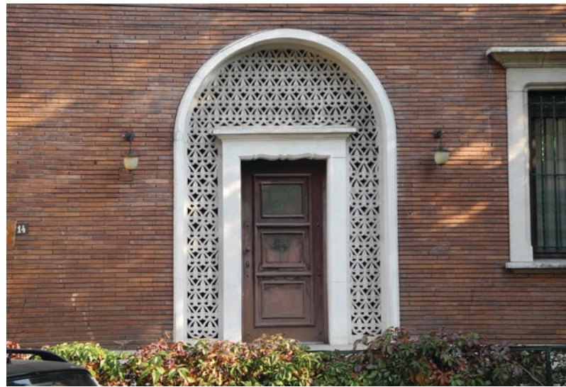
Fig.11. The main door of the building of Strada Athena 14. The brick facing, made by very thin elements and relatively thin joints, contrasts with the marble framing, of a rather classical style, of the openings. Exceptionally fine is the marble grid around the entrance door.
