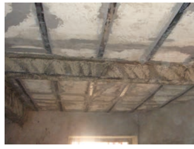
Fig.2.11 – Strengthening of RC floors with carbon fiber strips and fabrics
