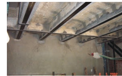
Fig.4.6 - Strengthening of reinforced concrete beams with carbon fiber strips
