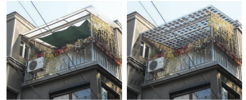
Fig. 12, 13 Bucharest, examined site. A simulation of the substitution of the canopy, made of glass or plastic, with a photovoltaic glass component.
