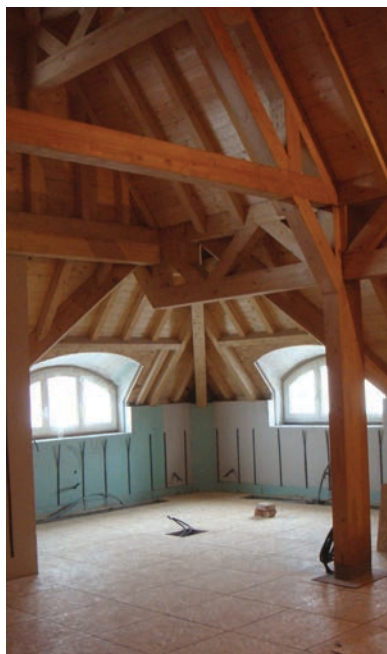
Fig.2.8 – New roof structure
