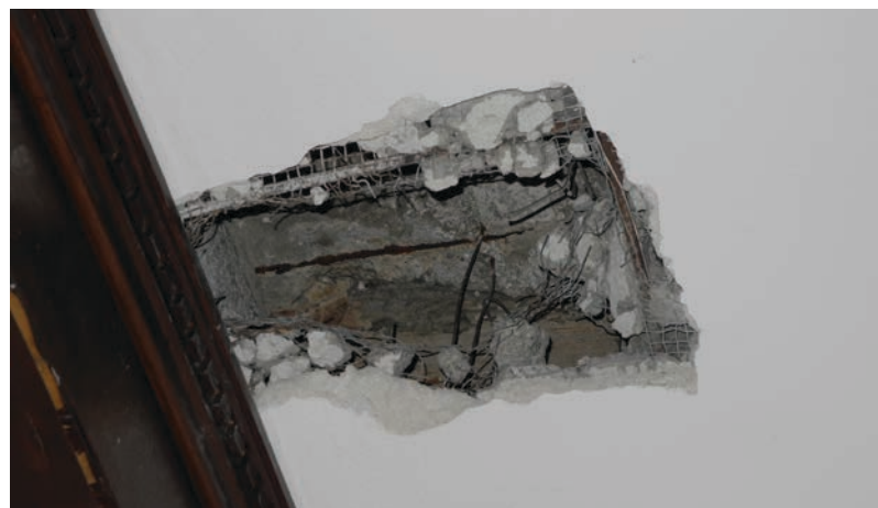
Fig. 9. Detail of the floor structure of the living room. The beam, in concrete, has been covered by wooden boards and enriched by moulding. The hole in the ceiling shows the real structure: plaster on iron net, suspended to the concrete slab.
