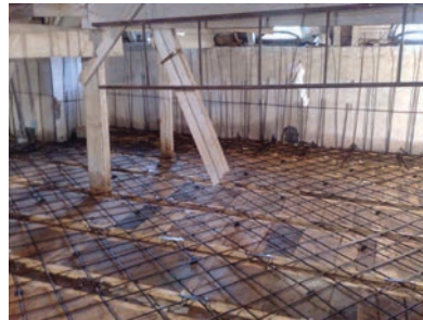
Fig.2.10 – Steel mesh for reinforced concrete topping on wood floor
