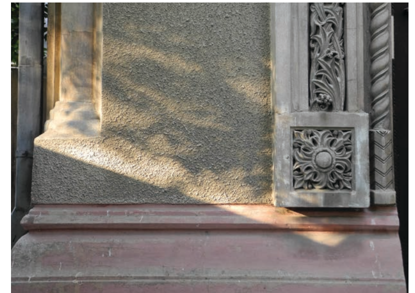
Fig.20. Particular with a rough render aside very elaborated columns and frames and basing on smooth colored moldings.
