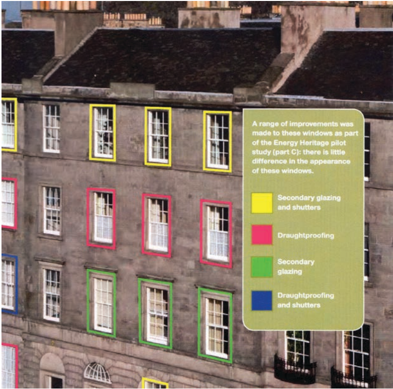
Fig. 6 Changeworks, Edinburgh World Heritage 2008. Energy Heritage: A guide to improving energy efficiency in traditional and historic homes. A range of possible interventions on traditional windows.
