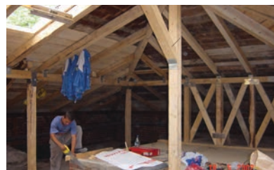
Fig.4.2 – Roof structure under rehabilitation
