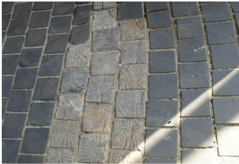
Fig. 5. The paving sections of tree trunk juxtaposed. Note the reintegration with similar elements.
