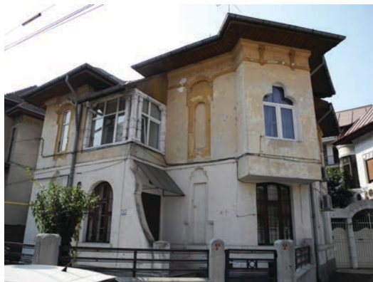
Fig. 5. Building with false openings of varying depths.
