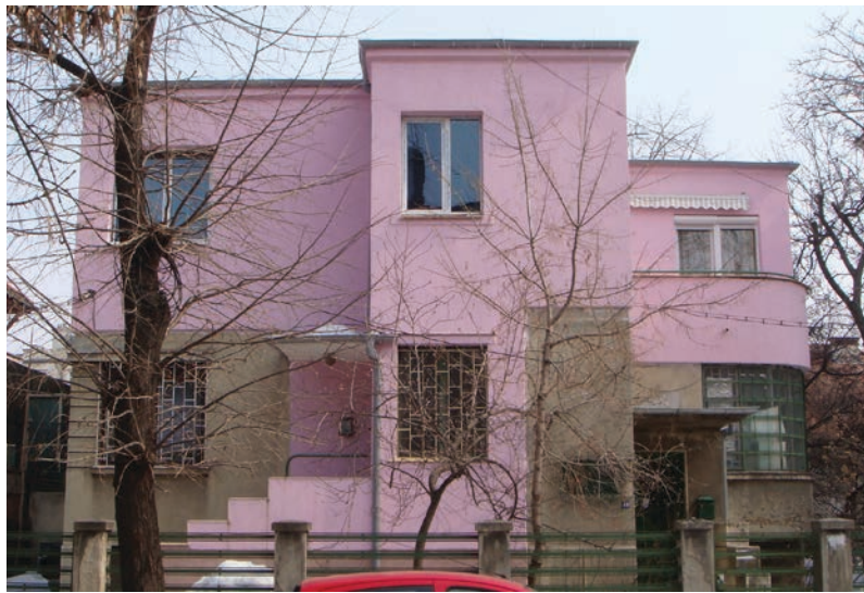
Fig.2. Thermal rehabilitation on Londra St: polystyrene and pink paint on façades.
