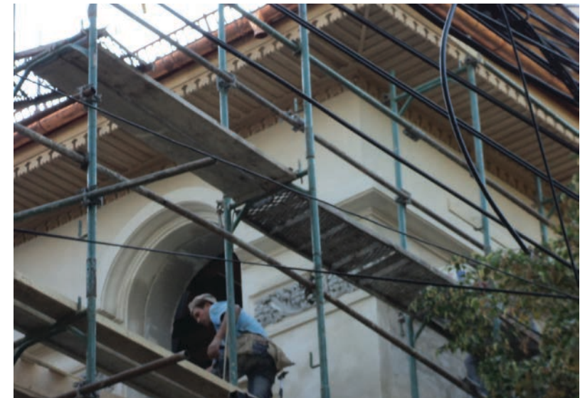
Fig. 4. Reproduction of original moldings.
