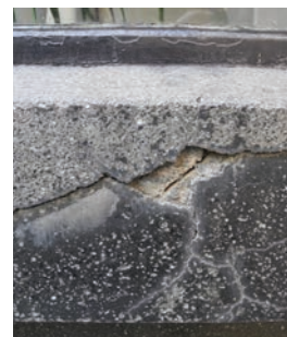
Fig. 27. Detail of the terrazzo cladding of the low fence wall of the building.
