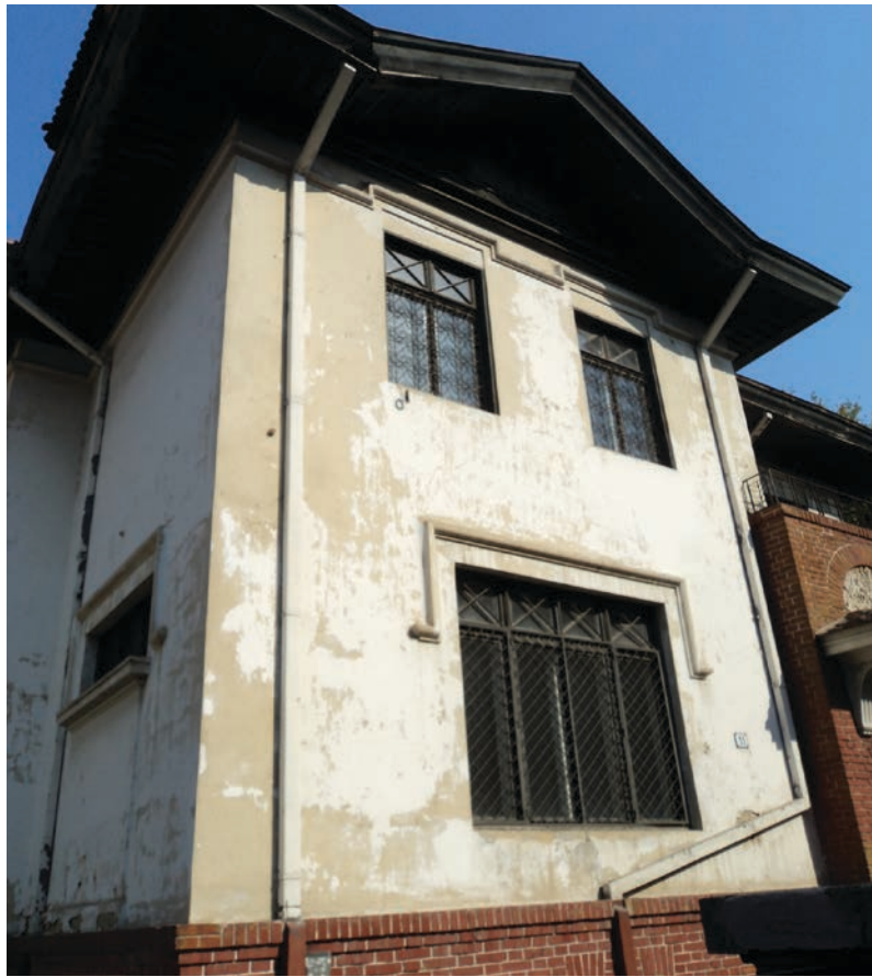
Fig. 5. Surface with a smooth finish; visible degradations only in the coating layer. Roofing with projecting eaves protecting the façades.
