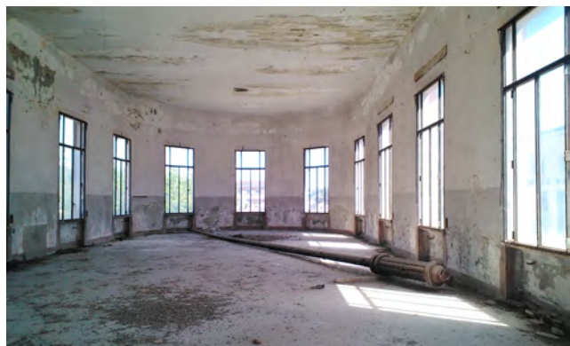
FIG. 3. Deleterious effects on the reinforced concrete floors of the seepage from the roof.
