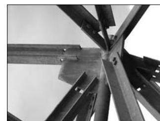
Fig 5B: Acoustic Barrier, ONL [Oosterhuis_Lénárd] 2004, File to Factory process of Mass-Customization generates 10.000 different nodes
