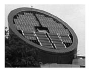
Figure 4. Roof-integrated photovoltaic and water heating evacuated tube solar collector installations at the ECOS Millennium Centre in Ballymena.
